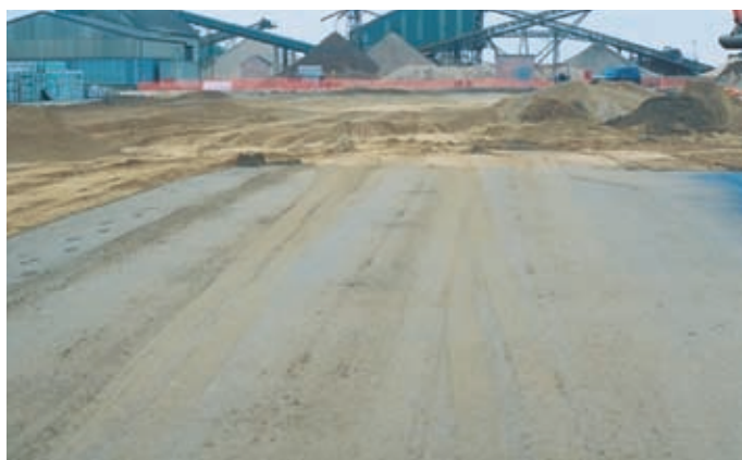
Figure 4: Mixture M2 after trafficking by loaded lorry
