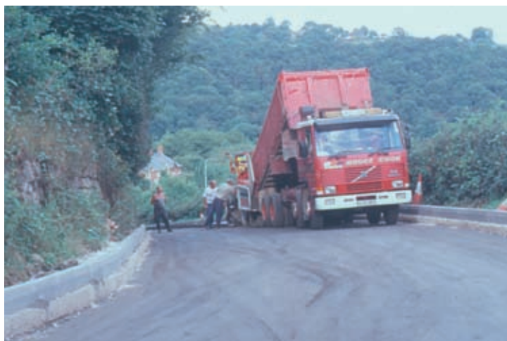
Figure 1: A52 Reconstruction, Staffordshire, 1997 – trafficking and overlaying fresh GFA subbase
