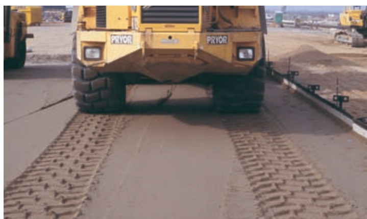
Figure 3: Mixture M1 showing significant surface disturbance under trafficking
